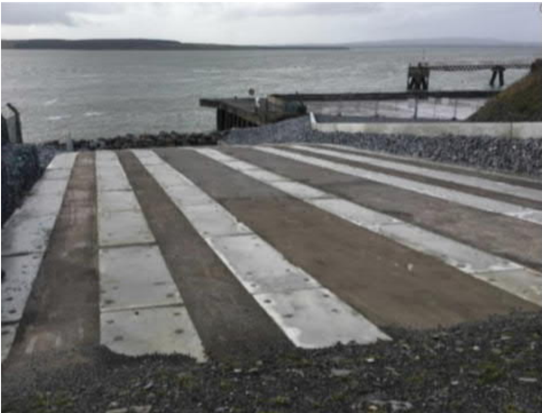
Figure 4.7: Typical Transition Joint Bay Following Final Reinstatement
