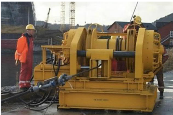
Figure 4.18: Example of a cable winch used during a cable pull-in
