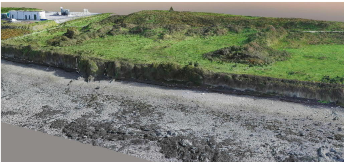
Figure 4.29: Aerial image showing the existing geology and topography at the proposed Kilpaddoge landfall
