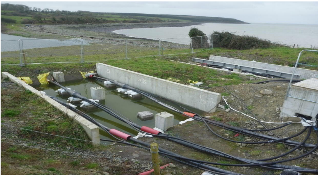
Figure 4.6: Typical Transition Joint Bay Before Final reinstatement
