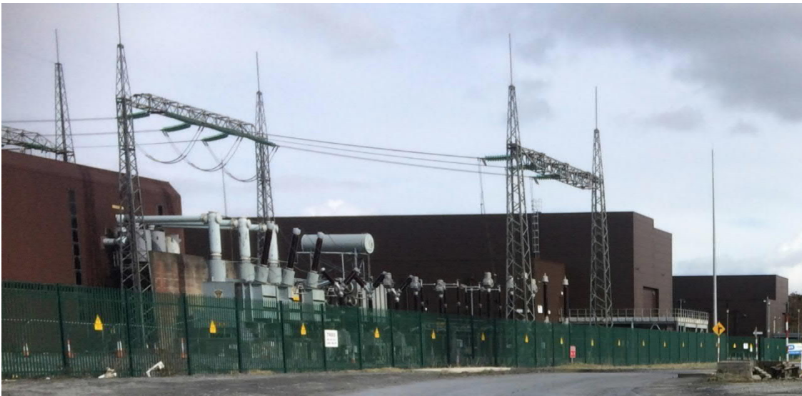
Figure 4.1: Moneypoint 400 kV GIS Substation Building
