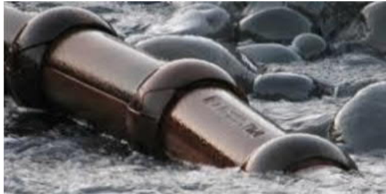
Figure 4.16: Typical cable protectors Articulated pipes
